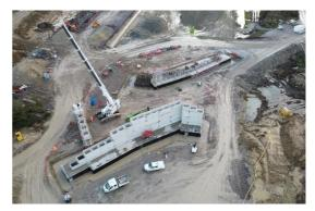
Precast concrete bridge abutments are installed at Station Road
